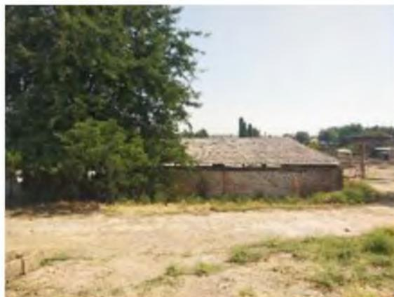
**Figure 39: Tashkent province. Old shelter with roof contained asbestos**
